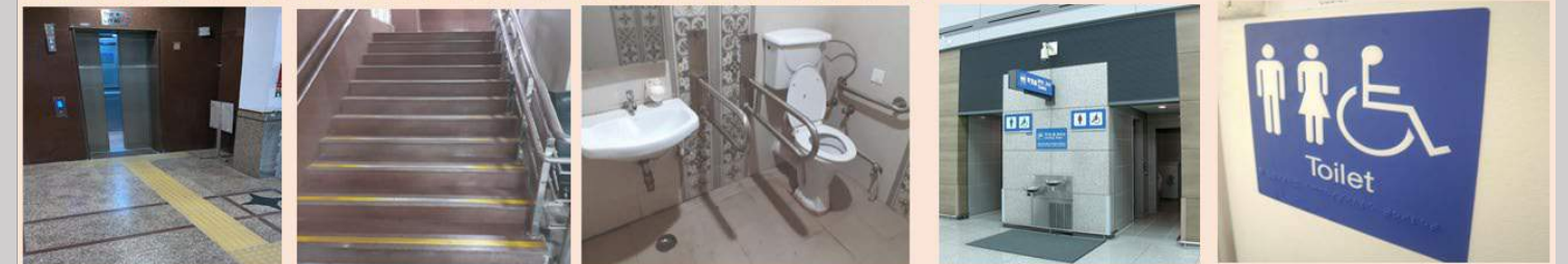
Lifts (Braille, Audio, Warning tile)
